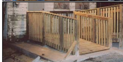
Top: Duane Breneman, Josh Brubaker, and Zach Galbraith work on a wheelchair ramp for a family in downtown Harrisburg Bottom: The wheelchair ramp.
